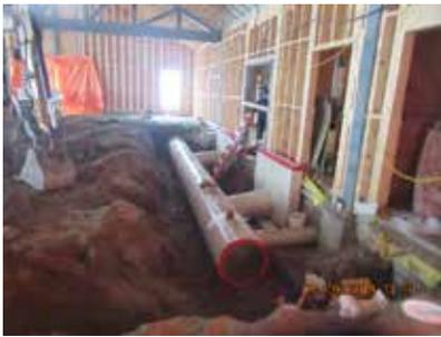
Crews are finished excavating in the gathering hall and have installed the fibre reinforced plastic (FRP) duct work to heat/cool the space. You can see some photos of the duct here on either side. The excavation is already backfilled with gravel and will be compacted and cement poured over top. The pour is scheduled for May 29th.
